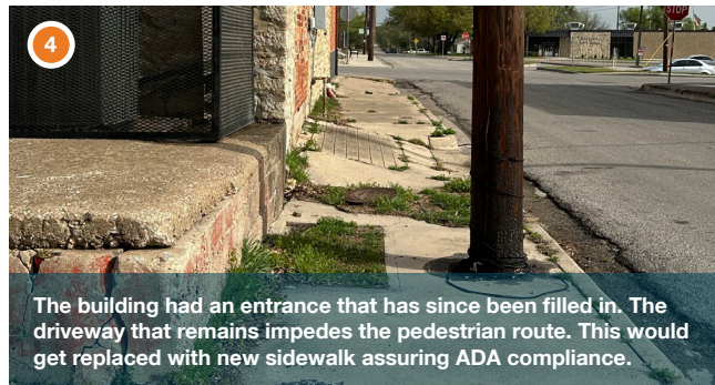
There are indications of subgrade failure under the existing pavement and #2 has non-compliant pedestrian facilities. We would evaluate the pavement to determine which areas will require full depth replacement versus mill and overlay. This solution will create cost savings for the City.
