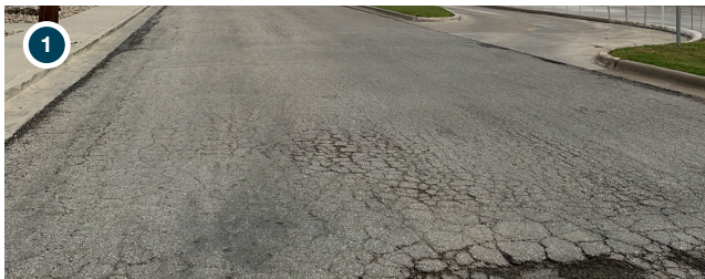
There are indications of subgrade failure under the existing pavement and #2 has non-compliant pedestrian facilities. We would evaluate the pavement to determine which areas will require full depth replacement versus mill and overlay. This solution will create cost savings for the City.
