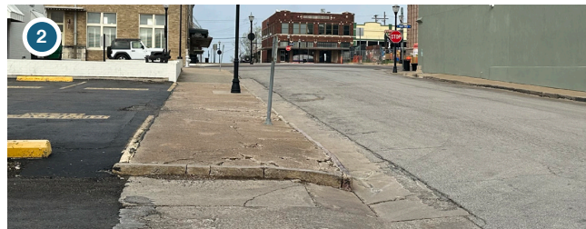
There are indications of subgrade failure under the existing pavement and #2 has non-compliant pedestrian facilities. We would evaluate the pavement to determine which areas will require full depth replacement versus mill and overlay. This solution will create cost savings for the City.
